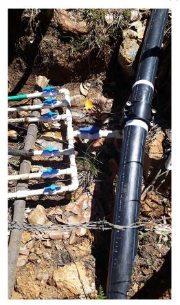
Figure 5 – Water distribution and outlet collar to "irregular" households in Bello Oriente from the communitarian pipeline
