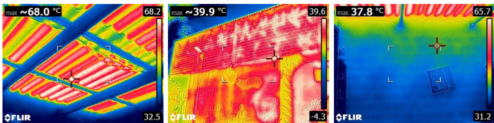
Figure 11 – Set of thermographic photos of house 4
