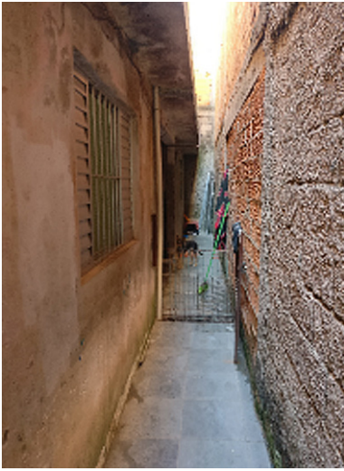
Figure 5 – House 7, uncovered side corridor
