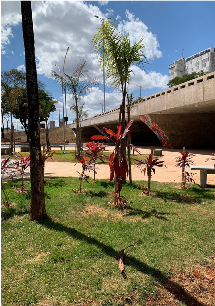
Figure 4 – View of the Central Viaduct of Brasília – 6/28/2021
