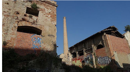
Figure 9 – Can Ricart power station, with the rooms that housed the steam engine and boilers
