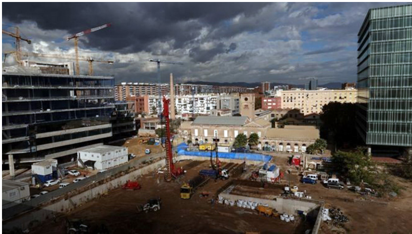
Figure 4 – Redevelopment work at Can Ricart
