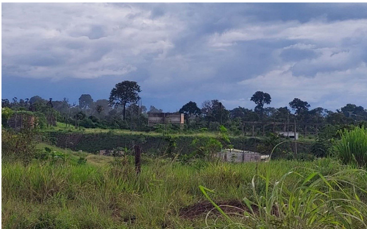
Figure 2 – Abandoned industrial structure overgrown with vegetation in MID, in 2022
