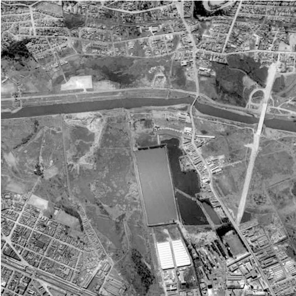
Figure 5 – Bridge of Santa Marina Avenue, 1958
