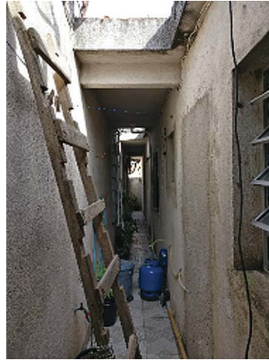
Figure 6 – House 9, partially-covered narrow side corridor
