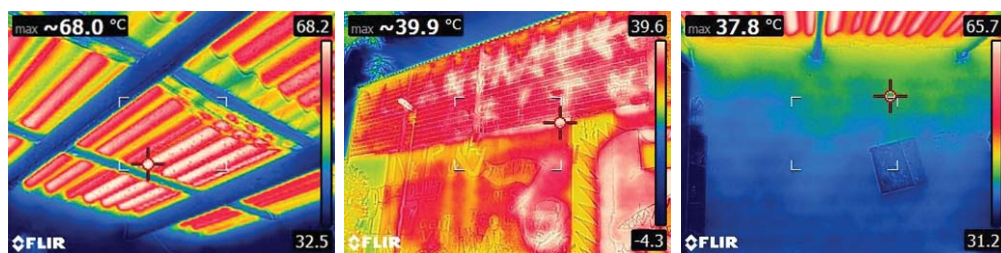
Figure 11 – Set of thermographic photos of house 4
