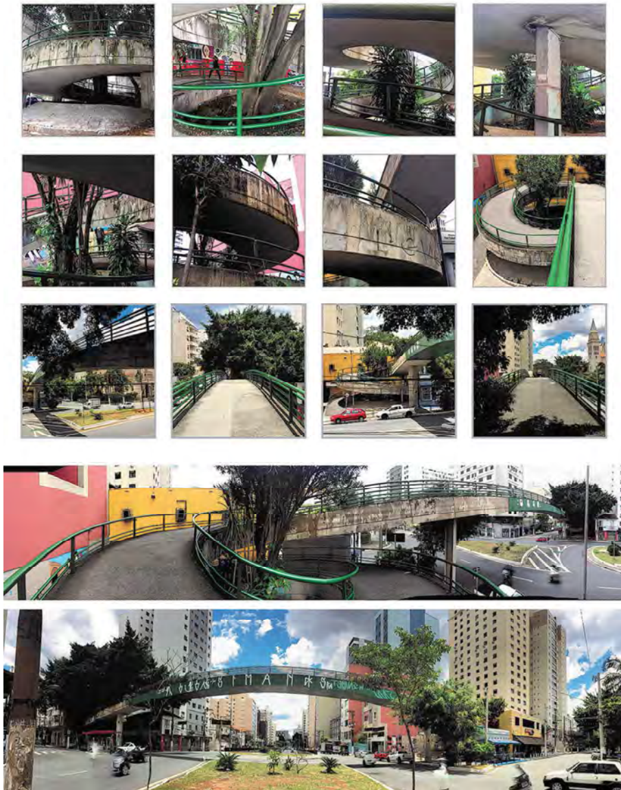
Figure 4 – Photos from the visit at Padre Pericles/Matarazzo walkway
