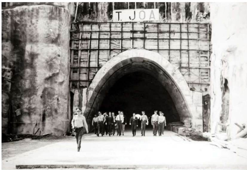
Photo 4 – Joá tunnel work, 1970s
