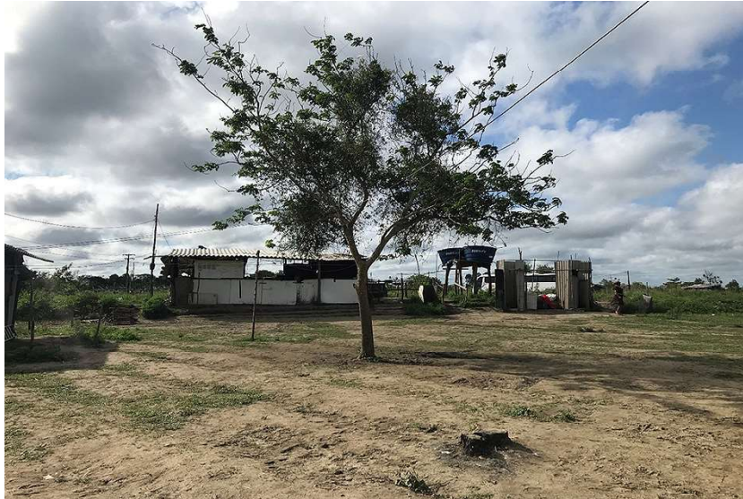
Figure 3 – The common kitchen, sinks and showers built by the encamped using surplus building material from the neighborhood
