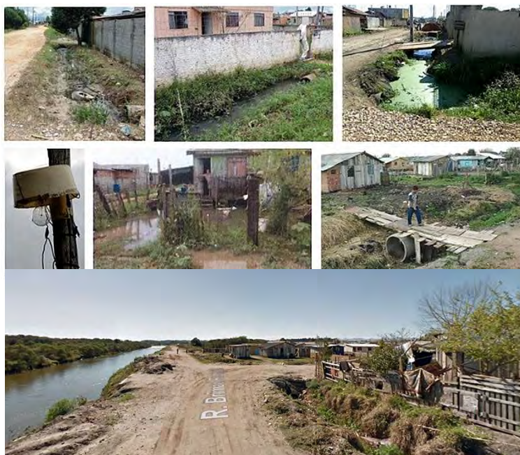
Figure 4 – Socio-environmental precariousness prior to the PAC works in Guarituba
