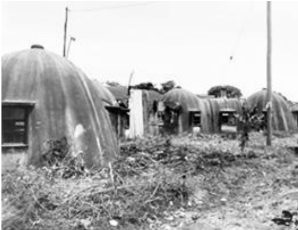
Figure 14: Bahati extruded concrete technology houses (author, 2013)
