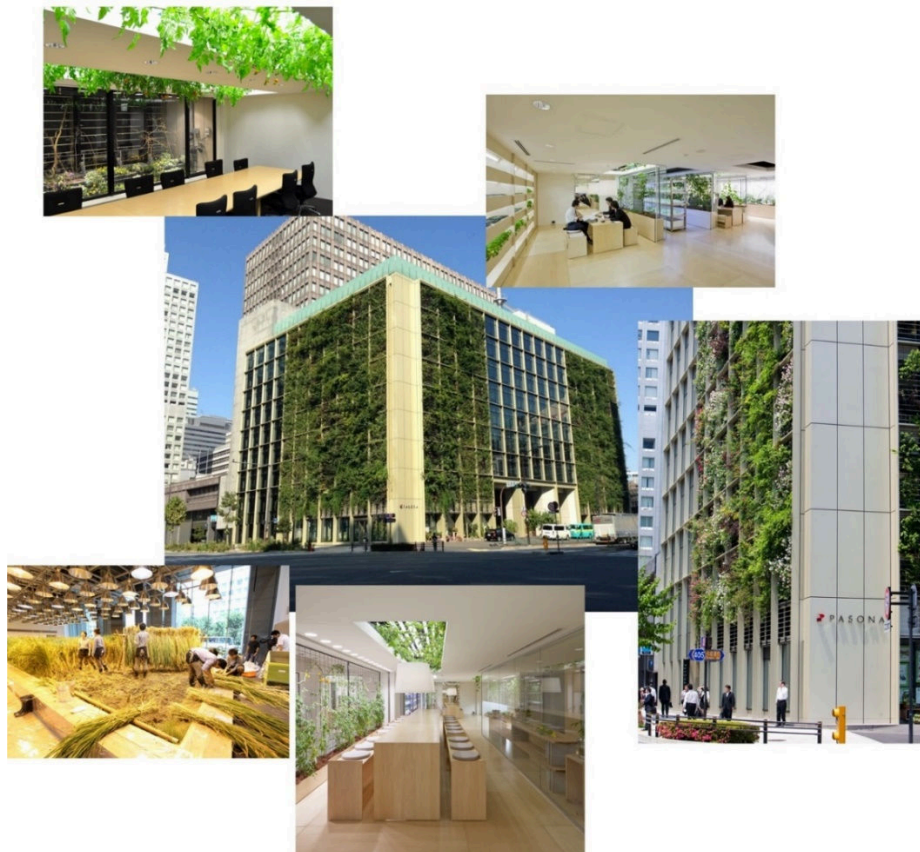
Figure 6 - Pasona VF building in Tokyo Japan
