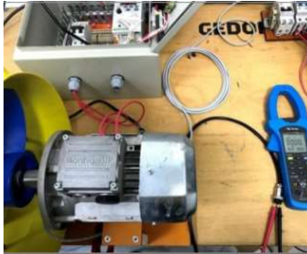
Figure 23 - Voltage acquisition as a function of generator rotation
