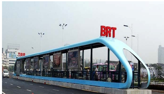
Figure 5 - Bus Rapid Transit ( BRT ) Station
